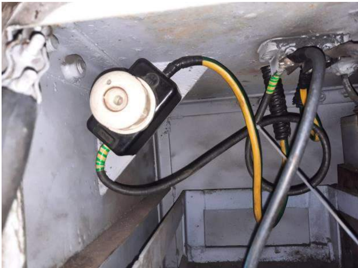
Photo no.22 – fuse assembled inside the niche of batteries.
