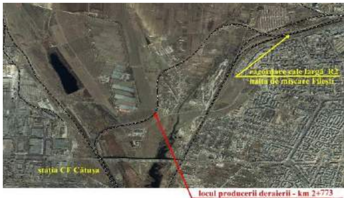
Figure no.1 Accident site
